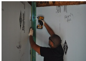
An AFSA member installs a corner brace for a Habitat for Humanity framing project
